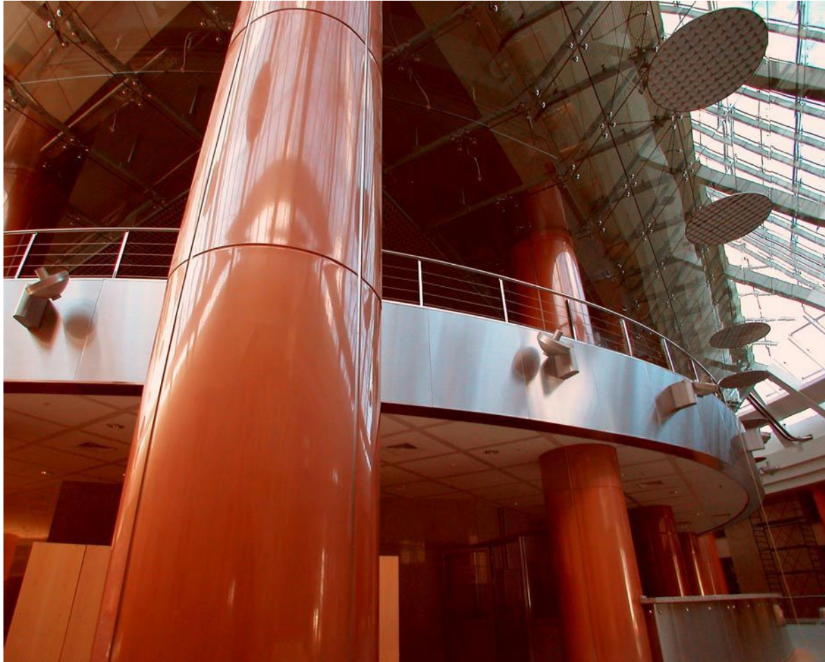
Italy – Commercial Building
