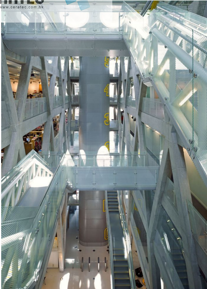
London – Commercial Building
